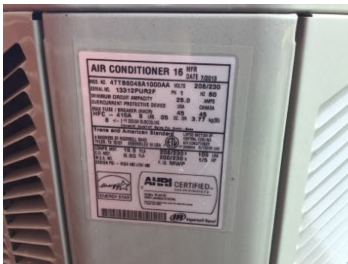
Condensing unit data plate
