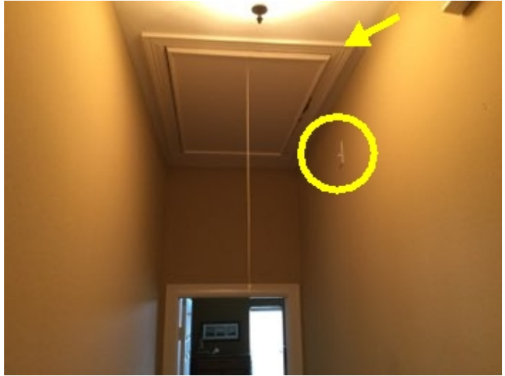
Attic access. Attic light switch
