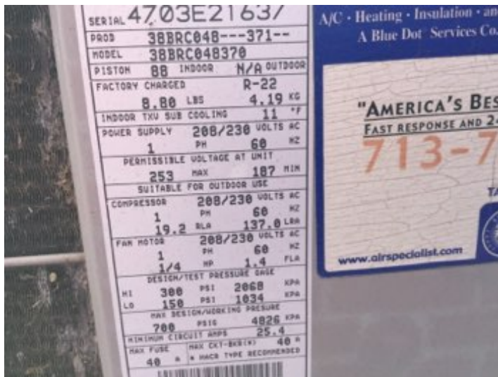
Condensing unit data plate
